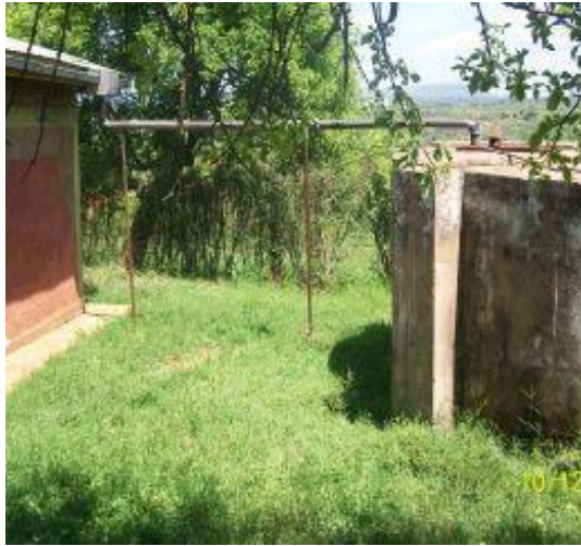
(a) Cement tank in Lembus Central
